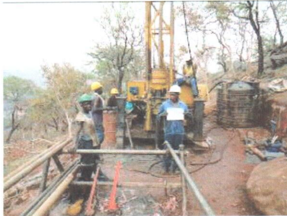
Figure 5 Le Badolite, Forage carottant
